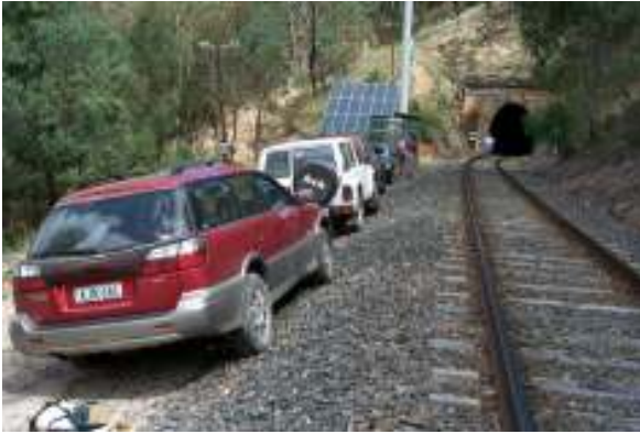
Carlos Gap tunnel east **.
